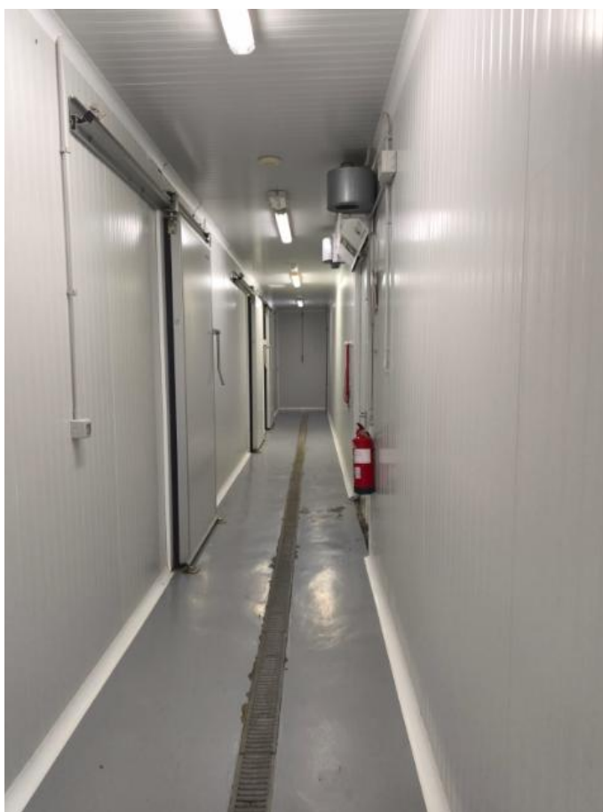
Figure 1. Insect rearing facility, with laminated insulated walls, resin floors and drainage for easy cleaning
